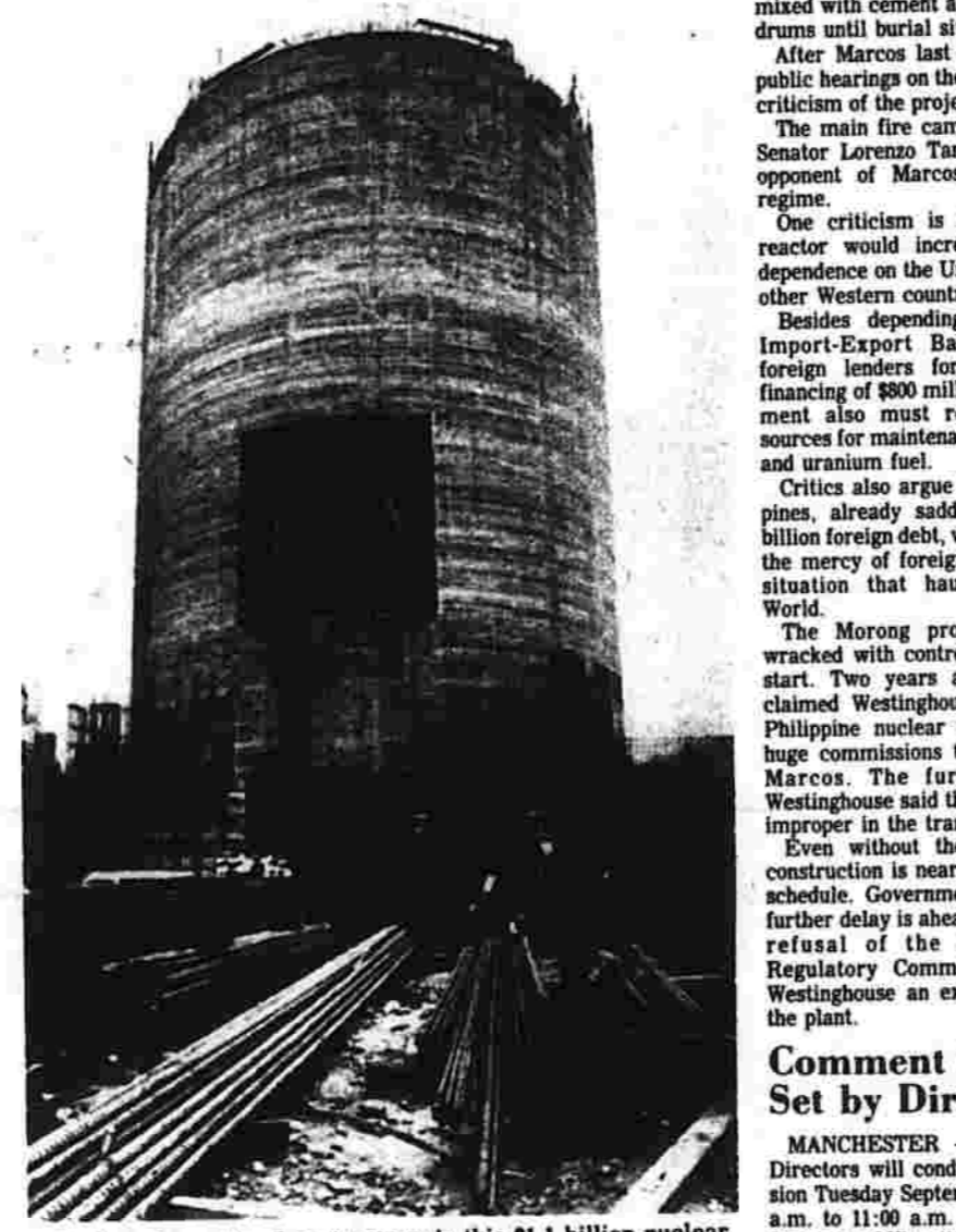
Center of a national controversy is this $1.1 billion nuclear power plant that Westinghouse Electric is building for the Philippines government. Work on the plant has been suspended by President Ferdinand Marcos because of his fear of a repetition of the Three Mile Island accident near Harrisburg, Pa. The plant lies between two dormant volcanoes, only 12 miles from an earthquake fault. (UPI photo)
